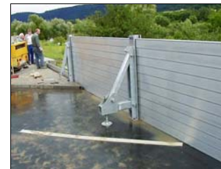
⑥ The Rear Buttresses can be assembled, if required
