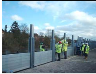
④ The Dam Beams are fitted between the Posts
