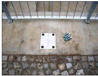
① The Anchor Plate is permanently cast into the Ground Beam foundation
