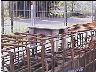
① The Anchor Plate is permanently cast into the Ground Beam foundation
