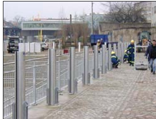
② The Supporting Posts are bolted to the Anchor Plates when the system is required
