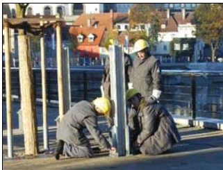
② The Supporting Posts are bolted to the Anchor Plates when the system is required
