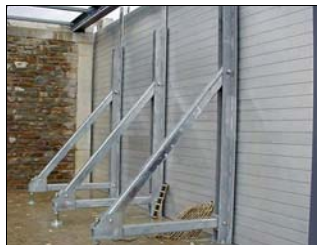
⑥ The Rear Buttresses can be assembled, if required
