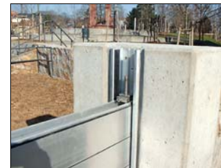
⑤ The Dam Beam seals are compressed with the Pressing Tool
