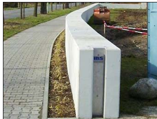
③ The End Supports are fixed at each end of the system
