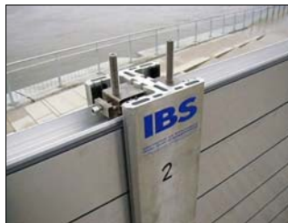
⑤ The Dam Beam seals are compressed with the Pressing Tool
